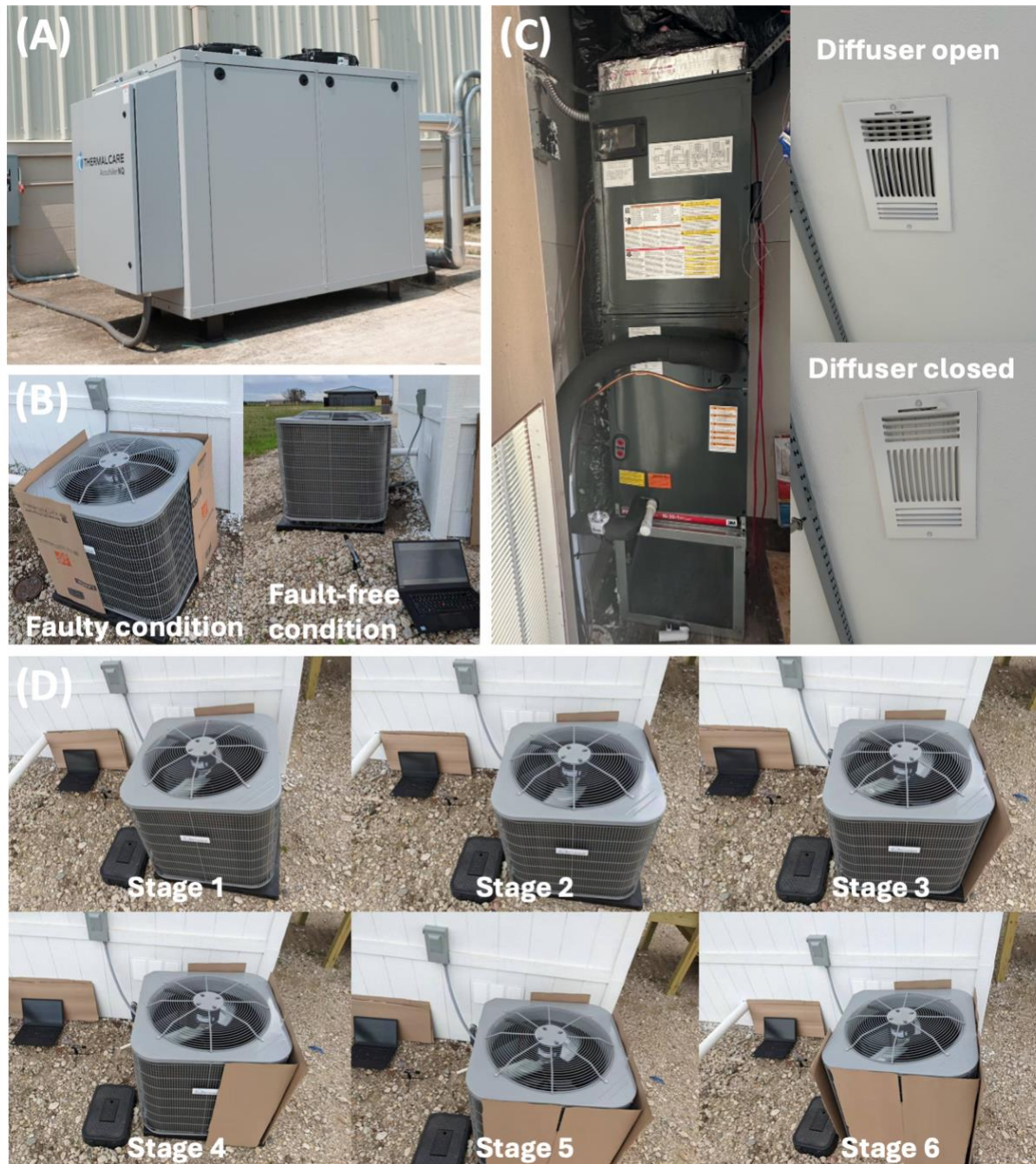
Figure 3: Acoustic data collected under various settings from (A) Air-source chiller; (B) A/C outdoor units; (C) AHU and Air diffusers; and (D) Condenser units.
